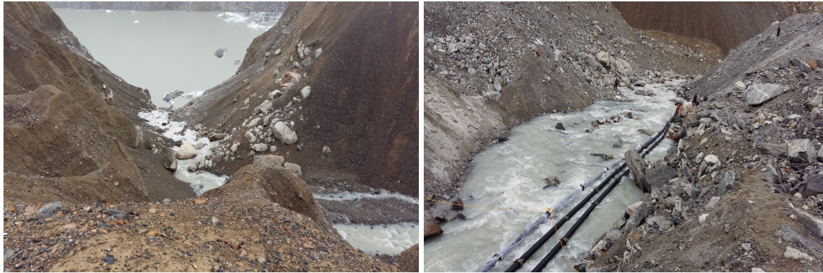
I. Photograph showing the outlet area of the lake and moraines dam & II. The photograph showing laying of pipelines with the help of rope in September 2016
