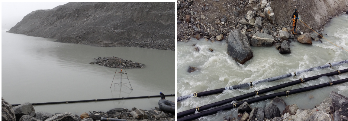
I. GLOF sensor installed in South Lhonak Lake & II. Pipelines laid down for the siphoning of water from South Lhonak Lake
